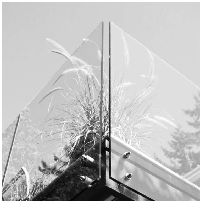
CODE REFERENCE: BAL-02 DESCRIPTION: Glazed Frameless Balustrade
