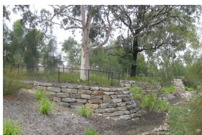
Figure 49: An example of fencing around a rock battered drainage channel.
