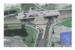
Sketch showing an artist's impression of a city-bypass built over a distribution roundabout with integral on/off ramps built into the abutments to take advantage of natural landform.
