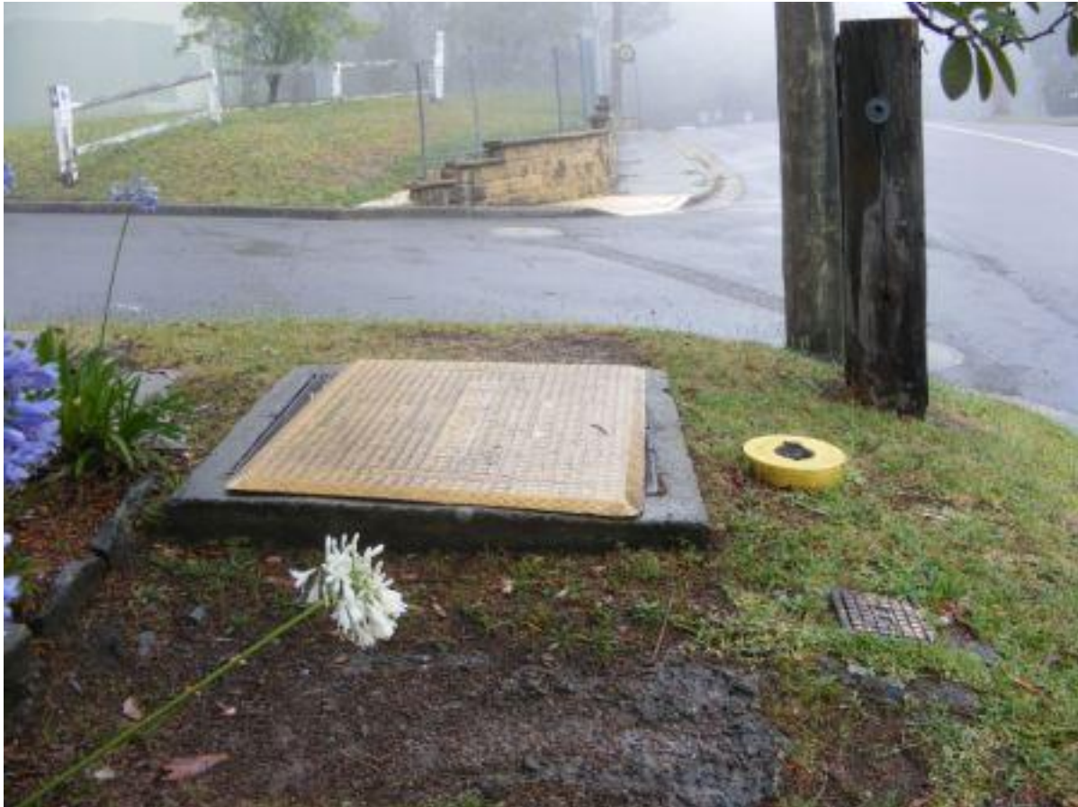
Figure 6. The northern verge of Grandview Road looking east showing large telecommunications pit right in the middle of the verge.
