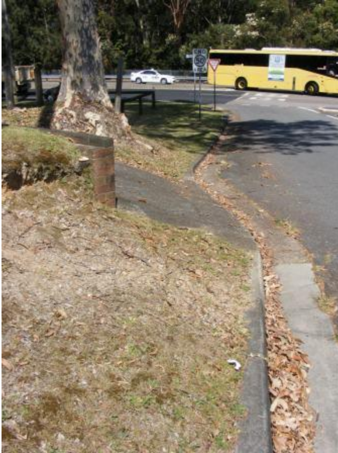
Figure 9. The northern verge of Grandview Road looking east showing a sloping gradient right to the edge of the kerb.
