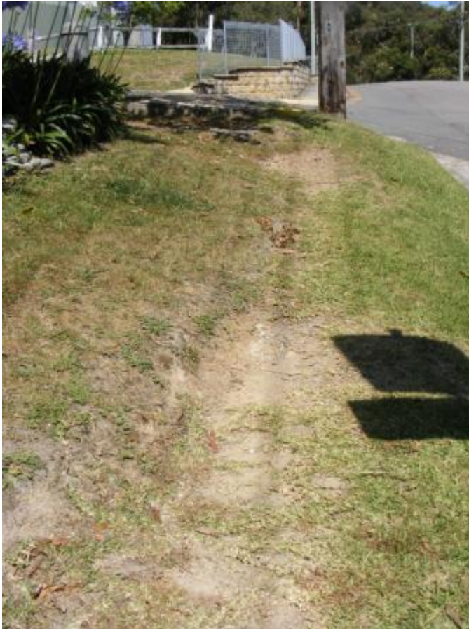
Figure 10. Northern verge of Grandview Road looking east and showing the uneven surface, sloping gradient and poor condition of the verge.
