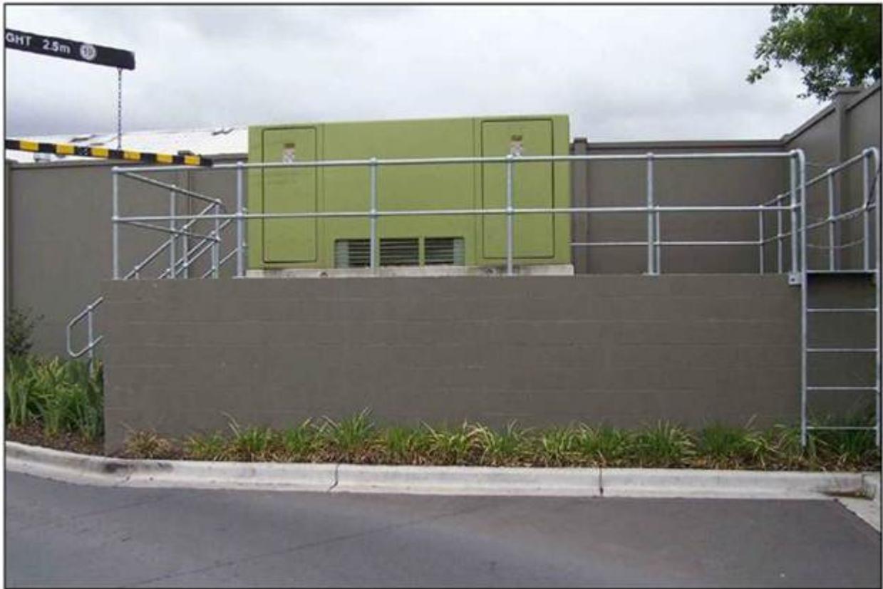
Figure 51 - Example substation raised above 1:100 flood level
