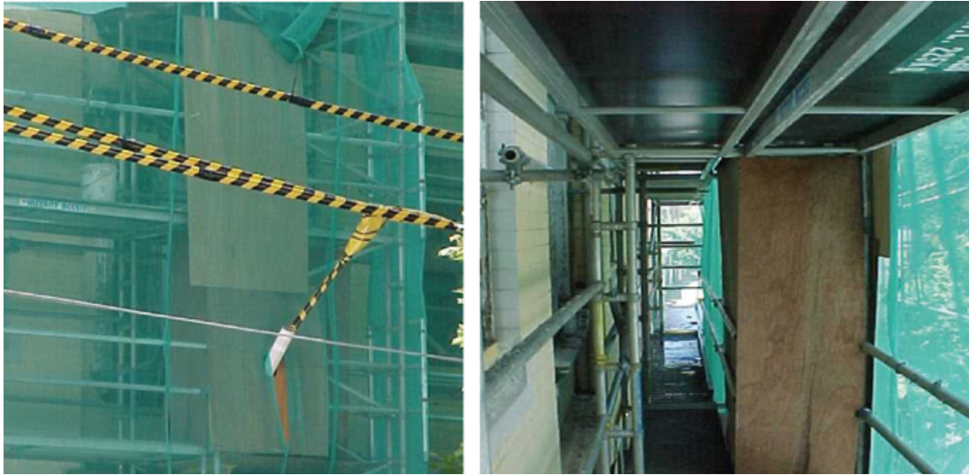
Figure 11 – Enclosure of overhead powerlines
