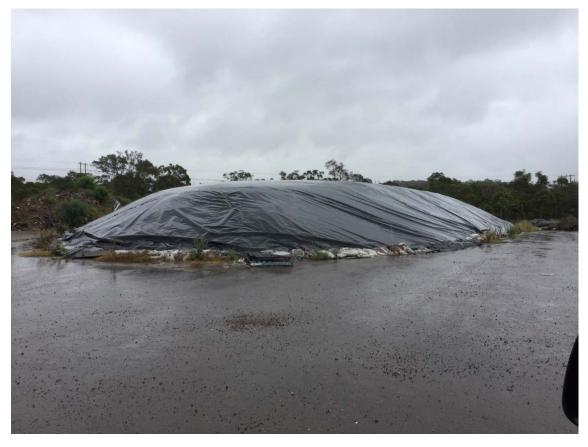
Figure 8 Typical External Stockpile – asbestos contaminated material
