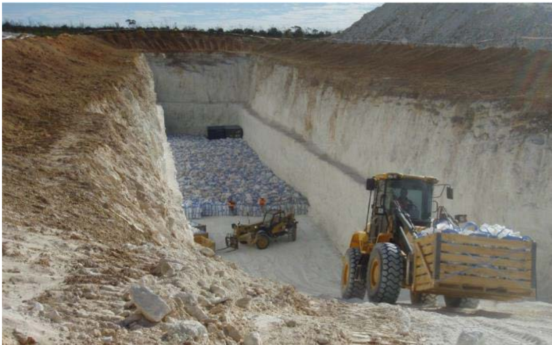
Figure 1 Example of an Australian near surface arid geological repository in thick, continuous natural clay bed with complete lack of water table.
