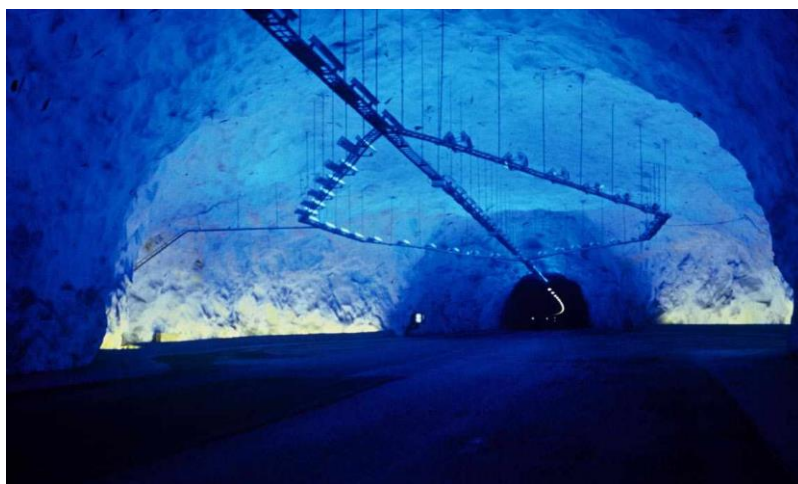
Image 1.6 – Image of the Lærdal Tunnel, Norway
