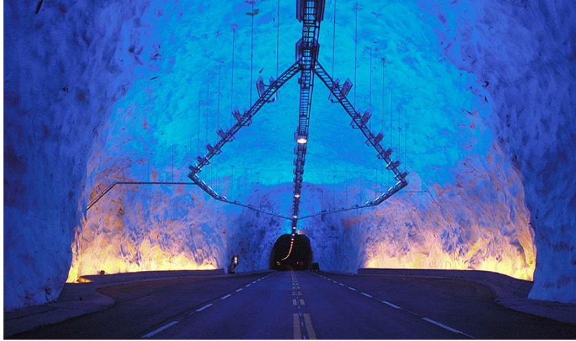
Image 1.7 – Image of the Lærdal Tunnel, Norway
