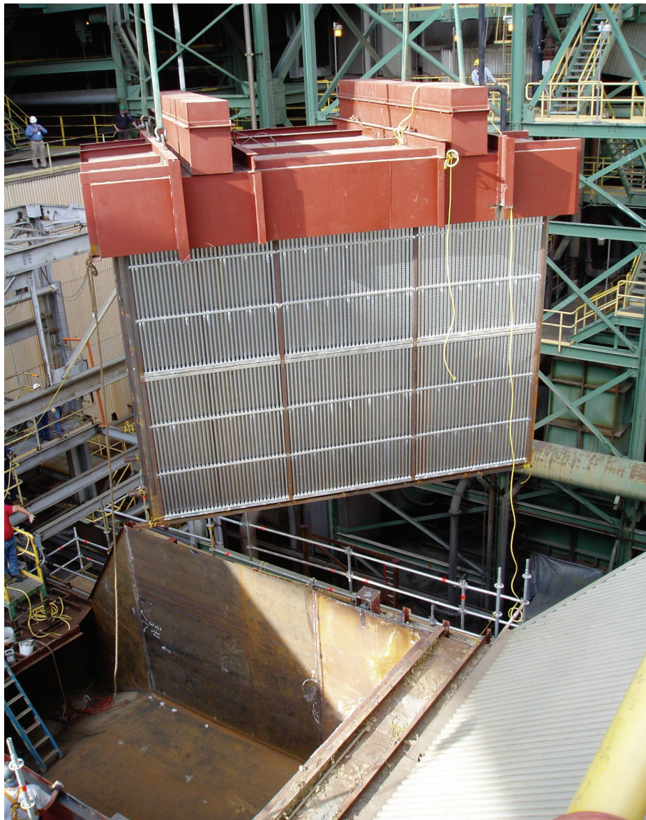
Figure 4: Agglomerator emitter arrays at Watson Power Plant USA
