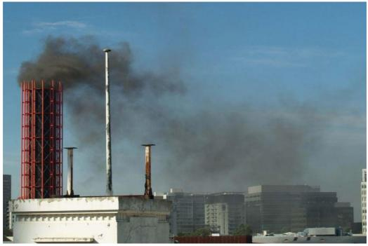
The fire in the Burnley tunnel was on such a day, the emissions were made visible by the addition of smoke, and the photo clearly shows that the surrounding area was fumigated. The tunnel pollutants are generally invisible, but they are deadly nevertheless.
