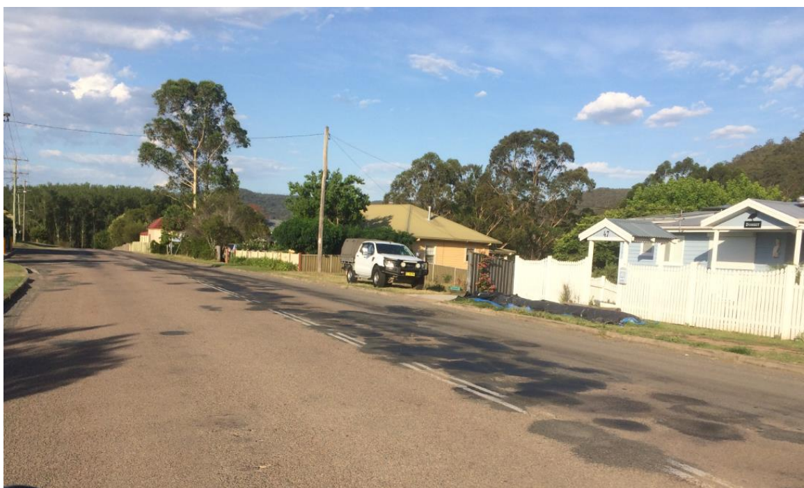
Photo 20– Pavement structural capacity inadequate – Tocal/Maitland Road Paterson
