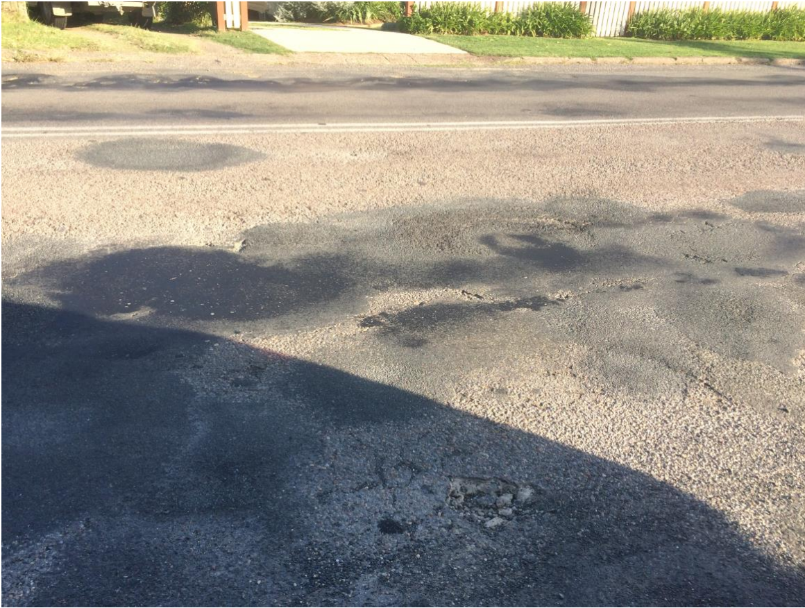
Photo 21– Pavement structural capacity inadequate Tocal/Maitland Road Paterson
