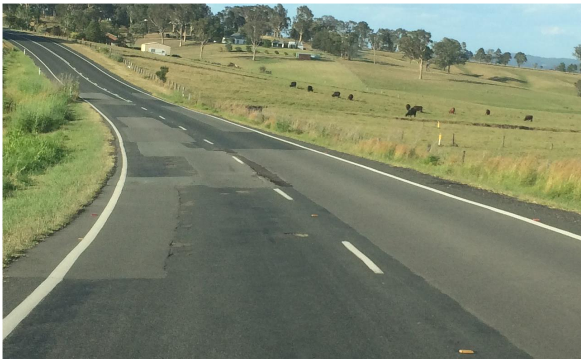
Photo 20– Pavement structural capacity inadequate – Tocal/Maitland Road Paterson
