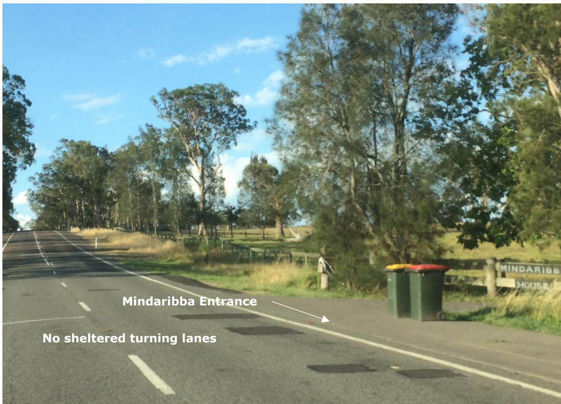
Photo 7 – Tocal Road and Lang Drive intersection (no sheltered turning lanes)
