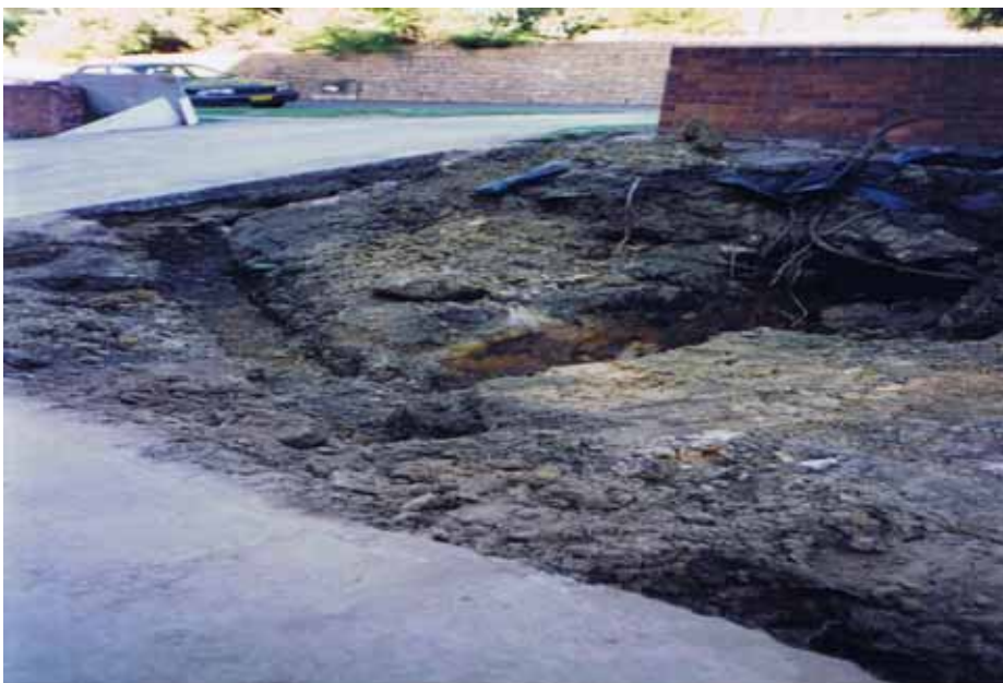
NO. 19 Preparing foundations for driveway brick wall and wider sweep of driveway
