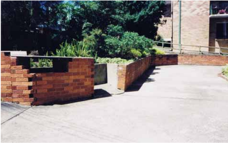
NO. 11 Before construction began with broken brick wall and leaning brick wall
