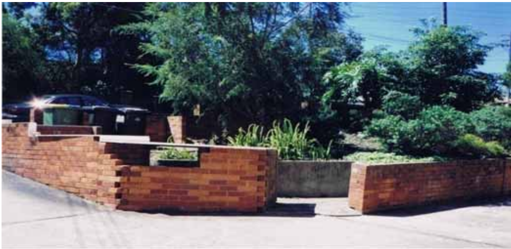
NO. 3 Before construction began with broken brick wall and leaning brick wall
