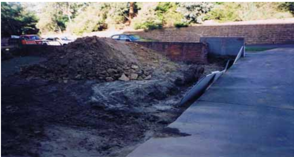
NO. 15 Preparing foundation of mail box brick wall
