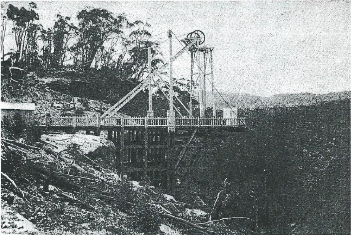
Ringwood Colliery platform and poppet head used to hoist coal up the cliff face 3
