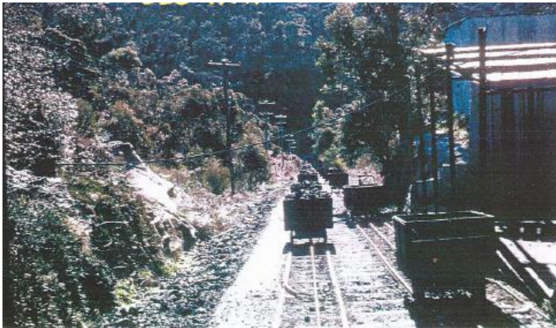
Inclined Tramway at Berrima Colliery showing full skips of coal being raised on the left track and empty skips being lowered on the right track
