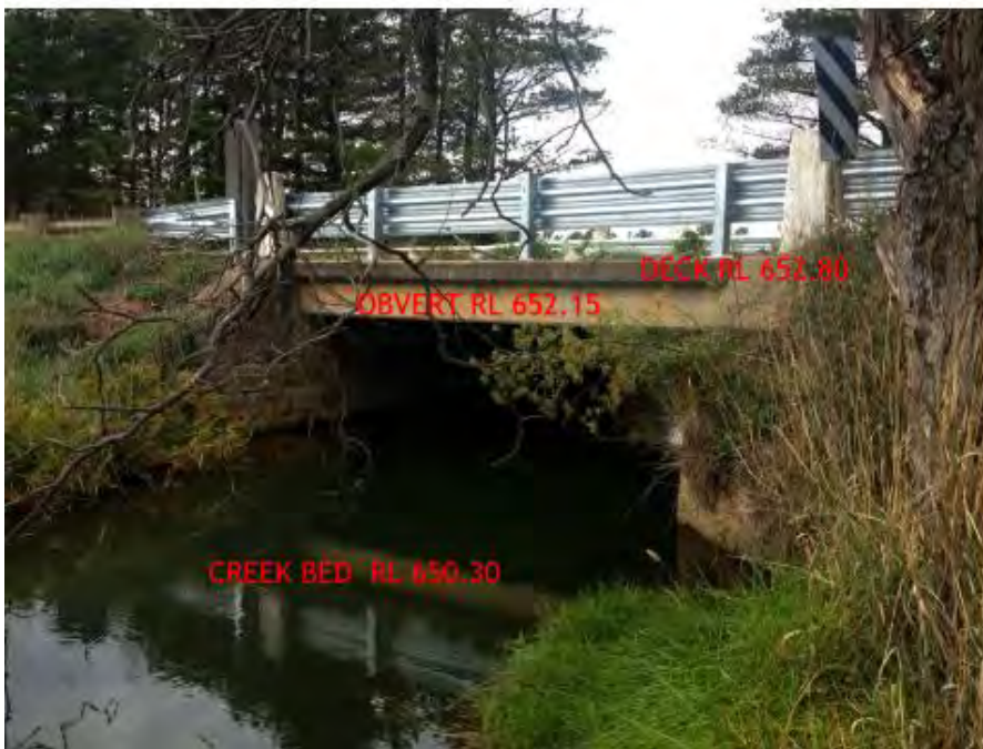
Photo 1.1 Old Hume Highway plank bridge
