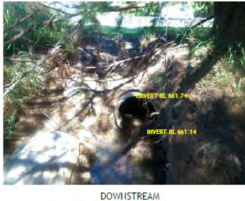
Photo 1.12 Photo of culvert structure under Berrima Road on the northwest tributary facing downstream
