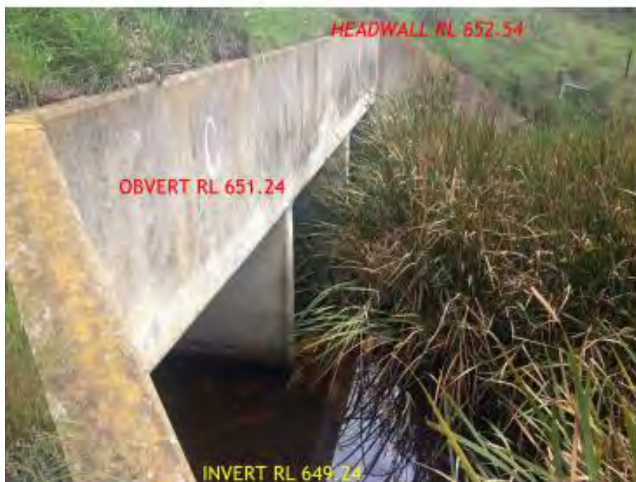
Photo 1.2 Hume Highway box culverts
