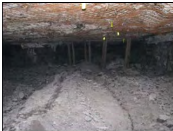
FIGURE 36. Moderate Floor Heave in 3-North Panel (outbye)
