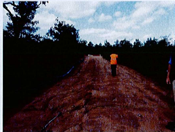
Plate 4: Bund wall forming northern edge of holding pond
