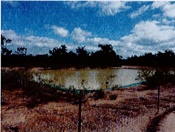
Plate 3: PVC lined holding pond
