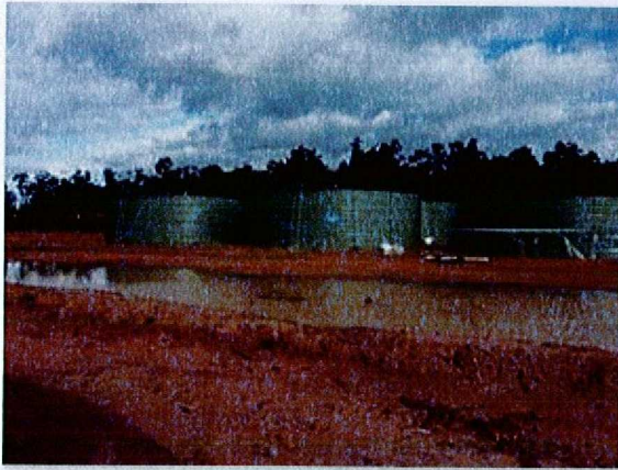
Plate 9: The six tanks with the partially completed tank to the right. Ponding within the low bund wall can be seen in the foreground
