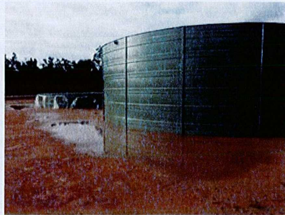
Plate 14: Ponding on the surface of the tank pad
