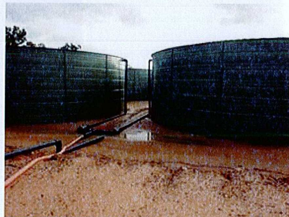
Plate 12: 'Lay flat' pipe entering the eastern most tanks
