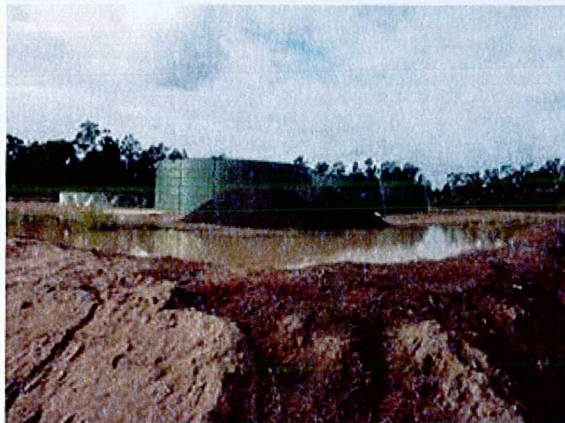
Plate 15: Looking north east showing ponding from bund wall and previous breach of bund wall
