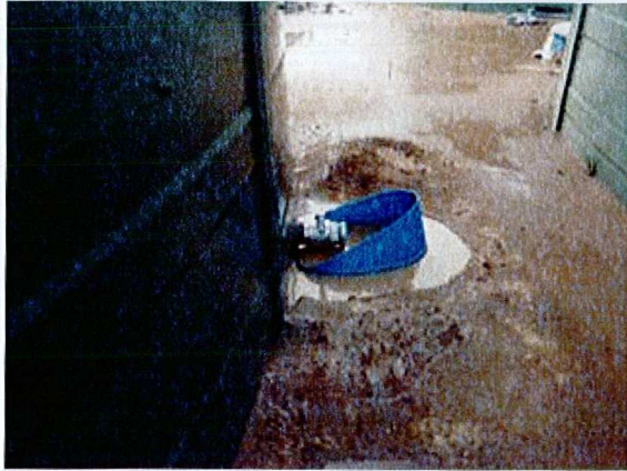
Plate 13: Leaking tank fitting
