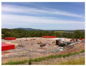
Photo 5.26 Fortuna multiwell pad after hydraulic fracturing of three wells and removal of most hydraulic fracturing equipment. Production equipment for wells on right side of photo. Source: Fortuna Energy, July, 2009.
