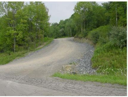
Photo 5.4 Access road and sedimentation controls, Moss 1, Corning, Steuben County NY. Photo taken during post-drilling phase. Access road at the curb is approximately 50 feet wide, narrowing to 33 feet wide between curb and access gate. The traveled part of the access road ranges between 13 and 19 feet wide. Access road length is approximately 1,100 feet long. Source: NYS DEC 2004.
