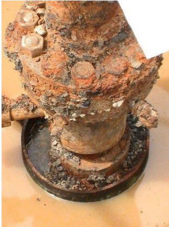
Example of one of the many corroding, crumbling Santos CSG wells in the Pilliga Forest
