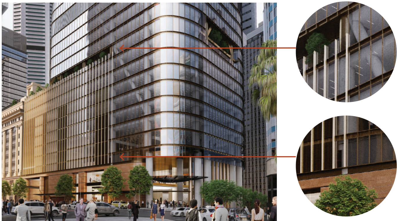
Figure 6 . Podium facade details vertical fins assist in resolving the transition from tower curtain wall glazing to the podium masonry base of 50 Martin Place
