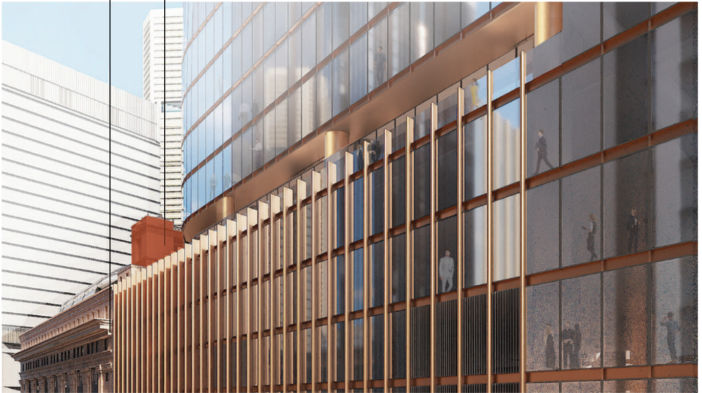
Figure 11. Detail of tapering vertical fins, recessed terrace and legibility of 50 Martin Place cornice and capital details
