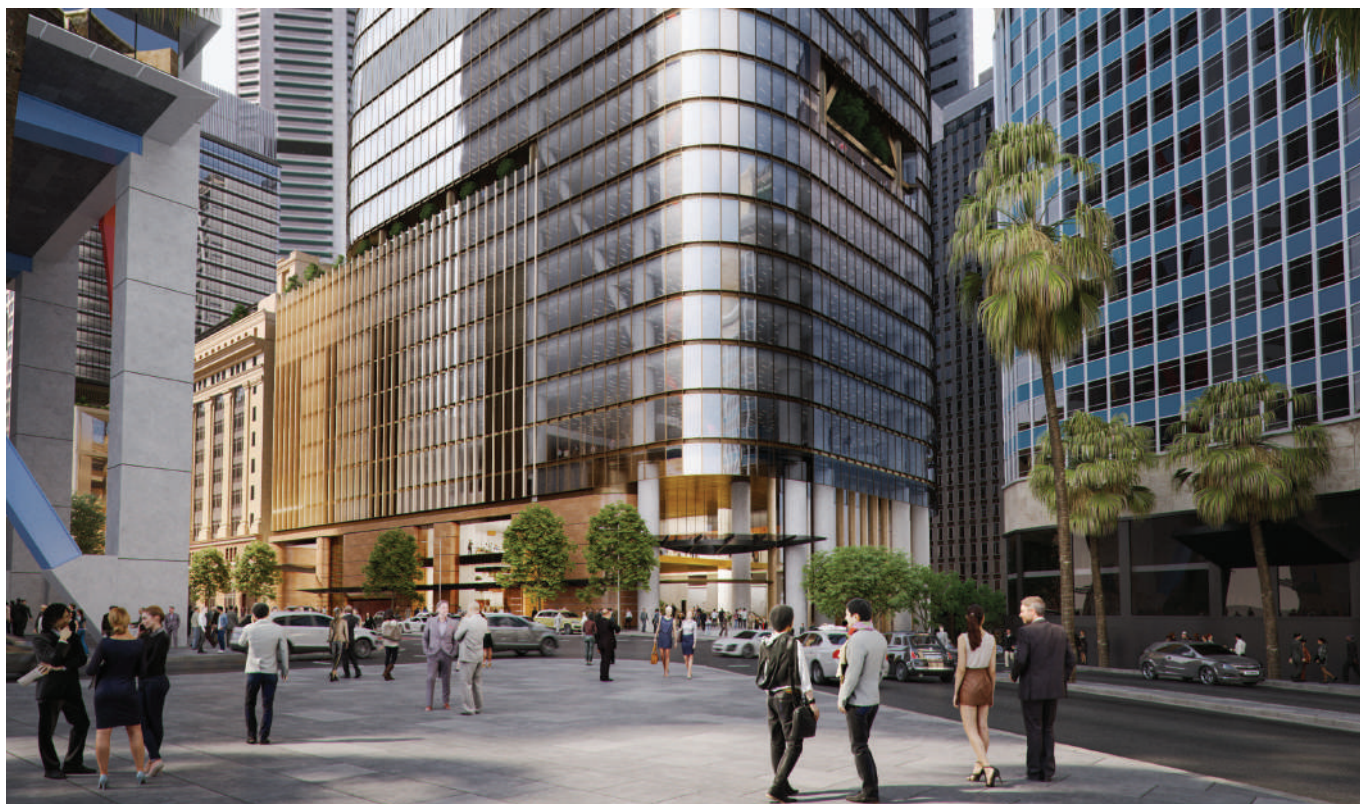
Figure 7. Vertical fins screen services ventilation requirements above the podium stone base
