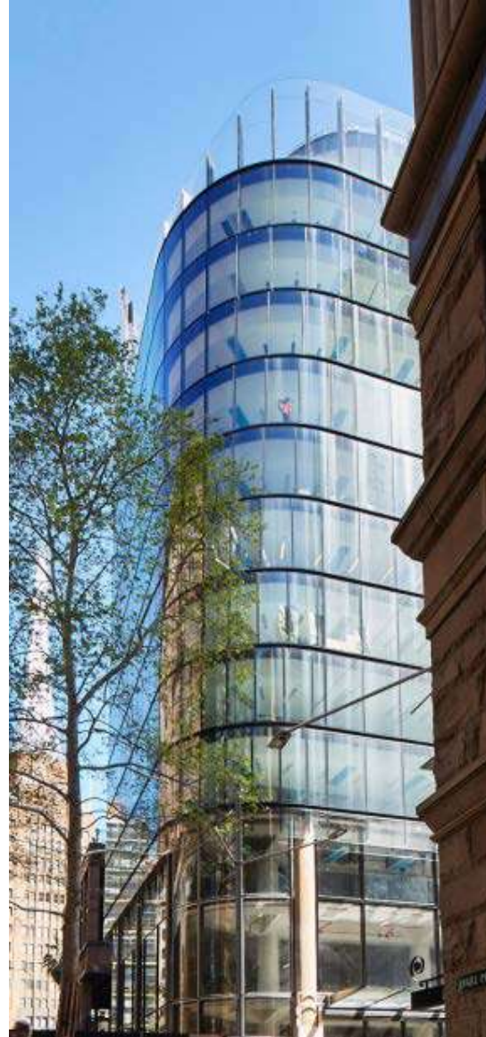
HIGH TRANSPARENCY LOW-E DGUs SOUTHERN "LENS" CASTLEREAGH ST LIFT SHAFT
