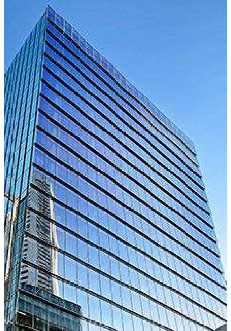
REFLECTIVE GLASS [MAX 20%] LOW-E DGUs TOWER GLAZING LEVEL 2 TO ROOF
