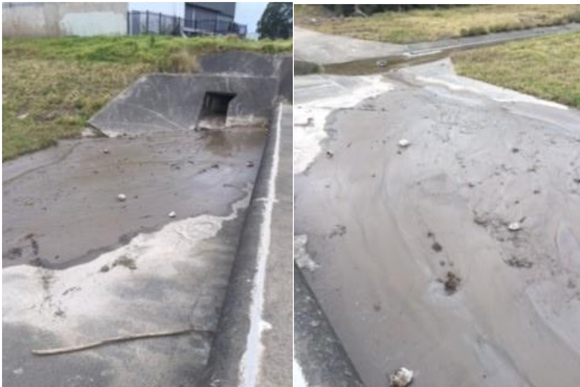
Figure 8 Sediment from the road in the stormwater drain and entering Bow Bowling Creek
