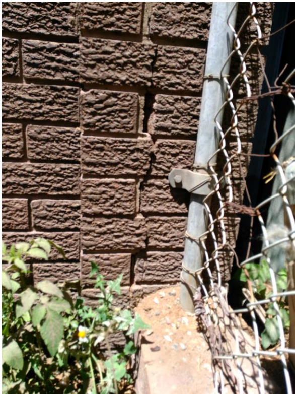
PLATE 7: Vibration damage to outside building wall at Unit 3, 35 Violet Street. Wall adjacent to Enviro Recycling
