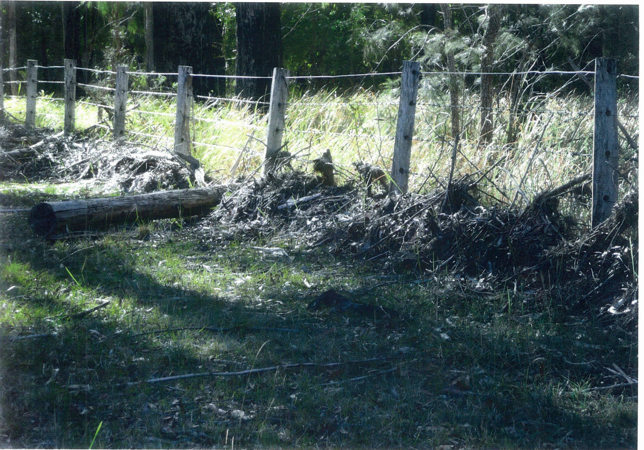
Flood Debris problems associated with fencing across creek floodplains
