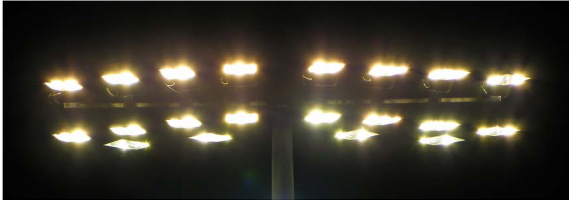
Figure 4. The head of one of four masts carrying full cut-off light fittings at the Victoria Oval in Dubbo. The illumination is of TV broadcast standard, but is confined entirely to the playing surface. (Wes Giddings)
