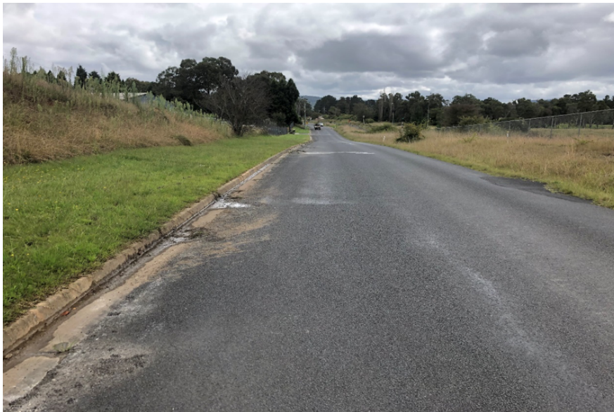
Lackey Road looking North from crest of hill on the road Note No Line marking and pavement failures
