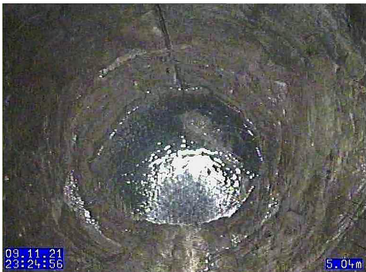
Figure 11 View of the bottom of Shaft 8 at the junction with the overt of the Bore
