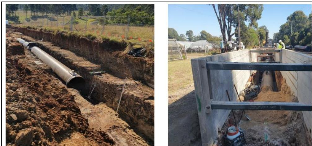
**Figure 2:** Excerpt from EIS. Typical underground pipeline construction method examples (benching (L) and shoring (R))
