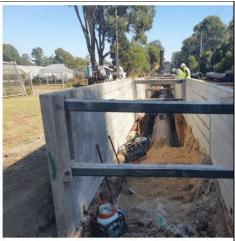
**Figure 2:** Excerpt from EIS. Typical underground pipeline construction method examples (benching (L) and shoring (R))
