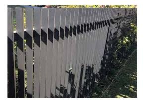
FENCE TYPE 2B-1200MM ALUMINUM BOUNDARY/ SECURITY FENCING.
