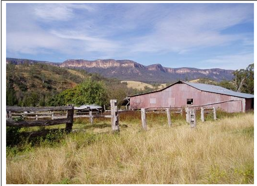
Figure 5: Joorilands shearing shed, historic pastoral property, Yerranderie State Conservation Area.
