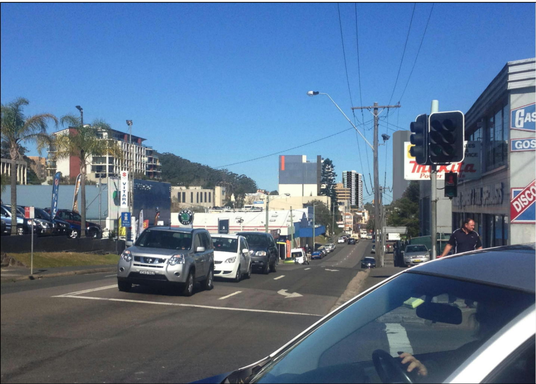
VIEW FROM NORTH AT CORNER OF ETNA ST AND MANN ST
