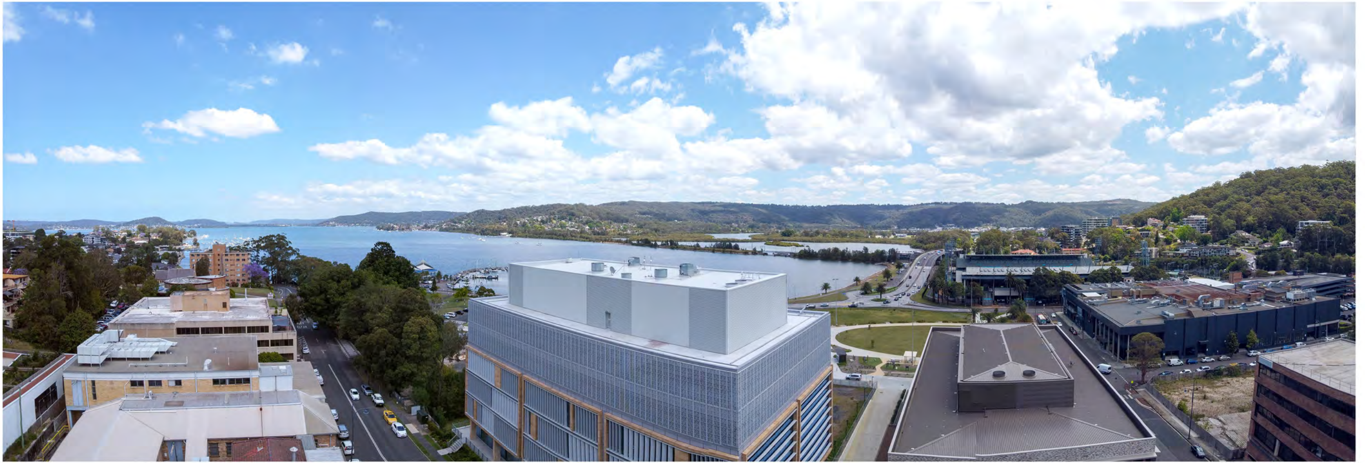
VP7 - existing photo - from residential level 7
