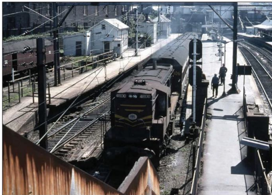
Figure 30: 1976 Locomotive 4104 hauling wiring train at south end of Redfern Station with single deck electric train in background [picture]. Note the precast concrete planks forming the surface of Platform 1, installed in 1956.
