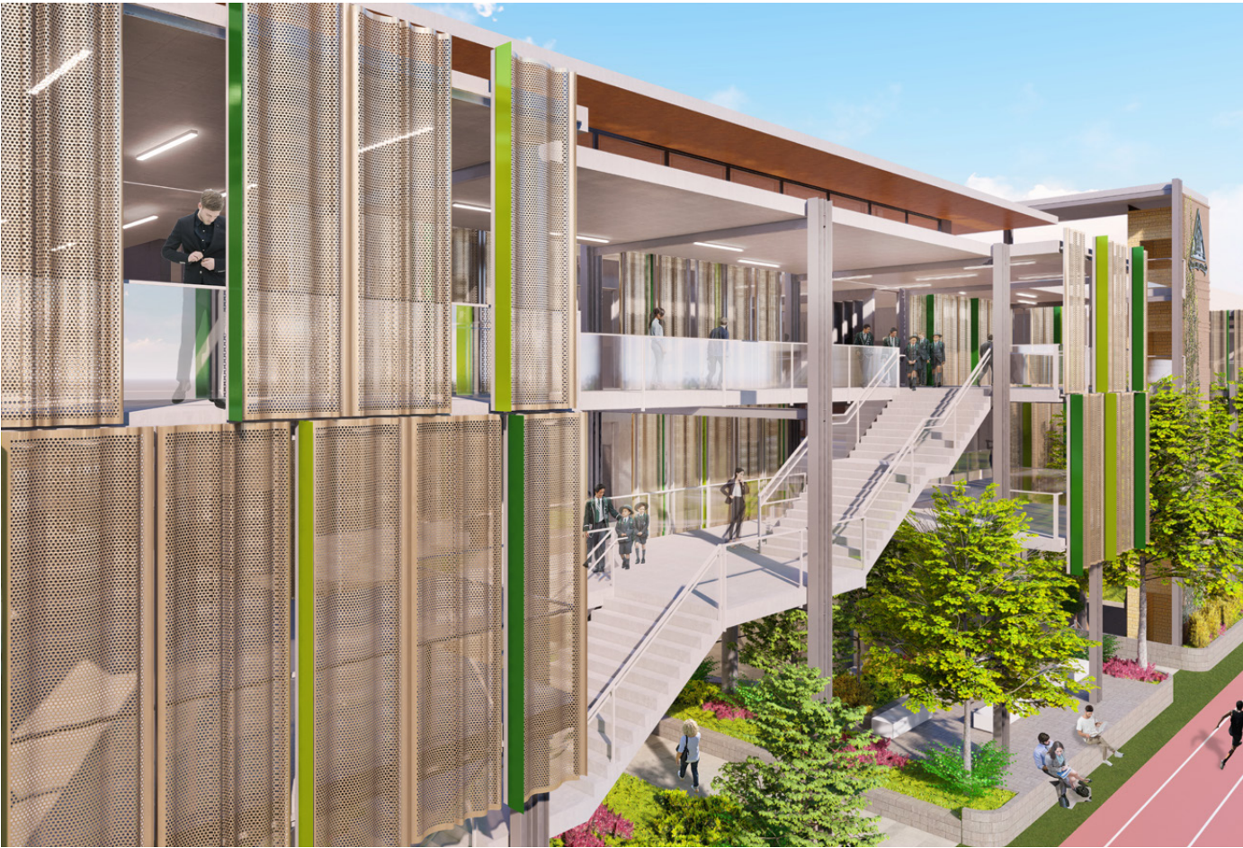
The combination of perforation of light weight screens, irregular install and layering all contributes to de-bulking the overall aesthetic of the Renewal Project.
