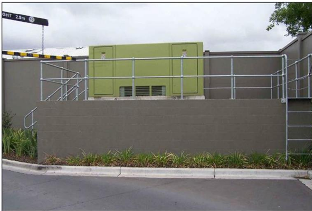
Figure 51 - Example substation raised above 1:100 flood level
