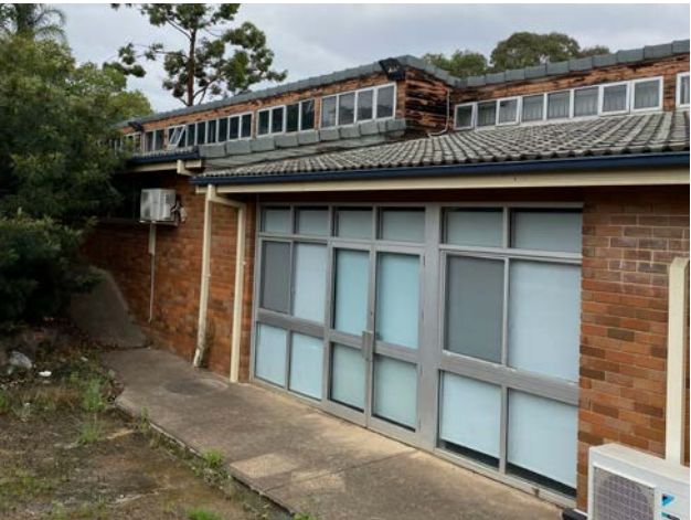
Substantial weathering to eastern highlights and cladding
