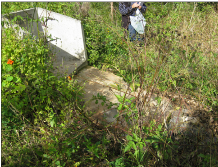
Photo 6: 450mm diameter Inlet pipe headwall and concrete apron. At approximate CH 65
