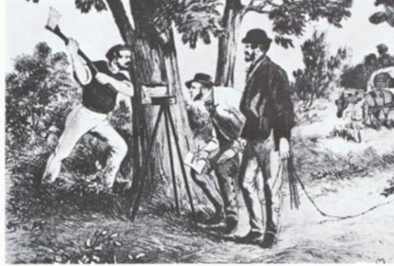
Fig. 1.4: Surveyors at work in 1865, using "metric" chain unit of 66 feet divided into 100 "links". Photo: Dept. of Main Roads, NSW.
