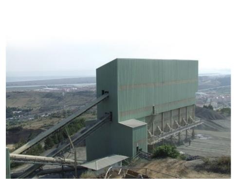
(crushing and screening plant is fully enclosed to minimise noise and dust)
