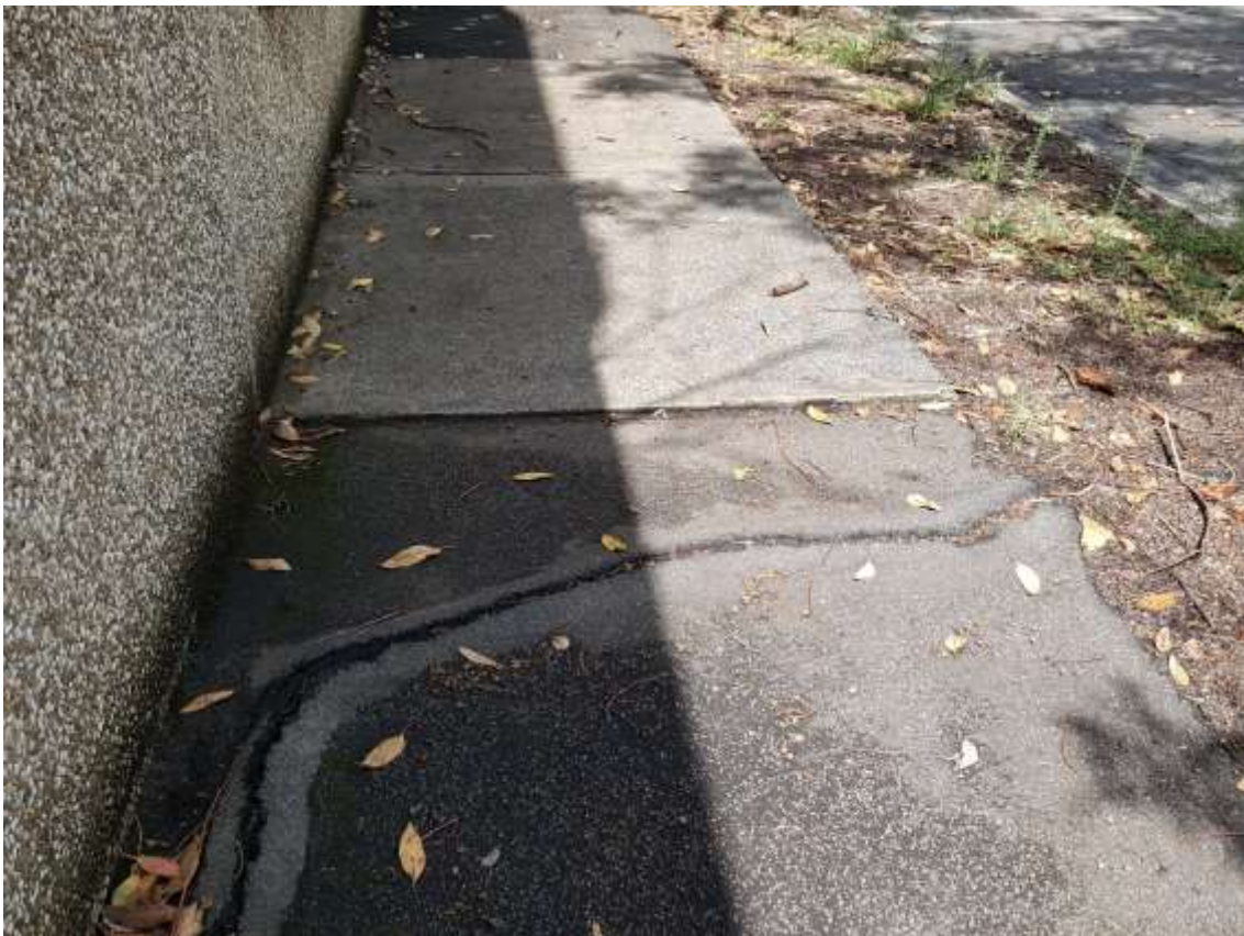
Photograph 12 – Tree 3 damage to path adjacent
