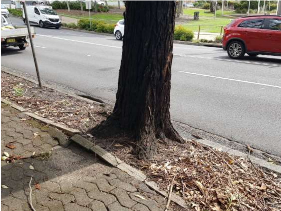
Photograph 19 – Tree 7 damage to pavement
