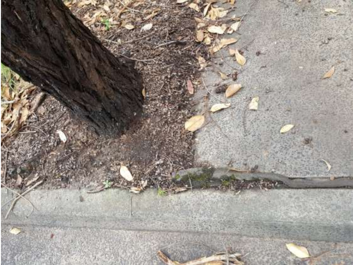
Photograph 5 – Tree 1 root between path and kerb
