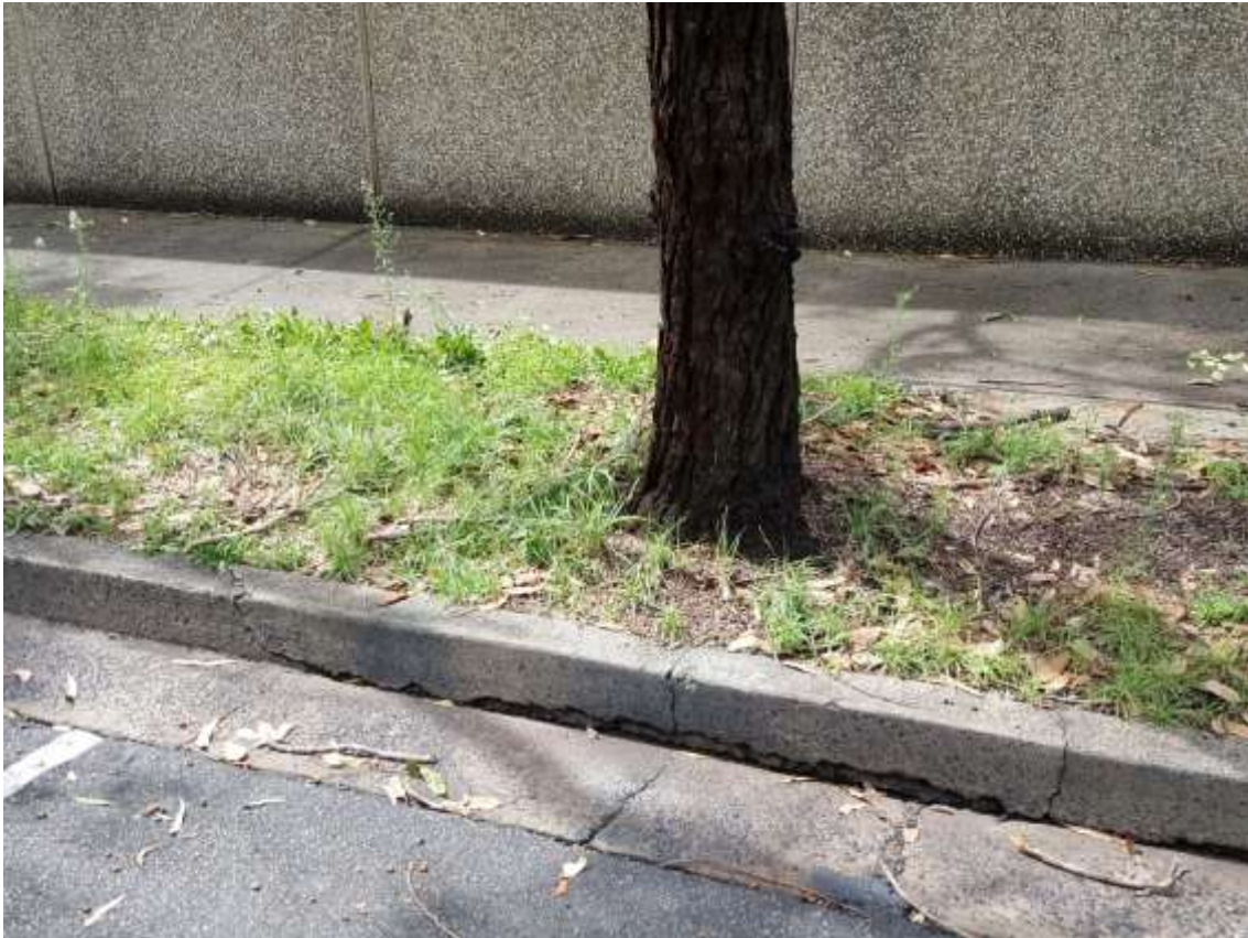
Photograph 13 – Tree 4 damage to kerb and gutter
