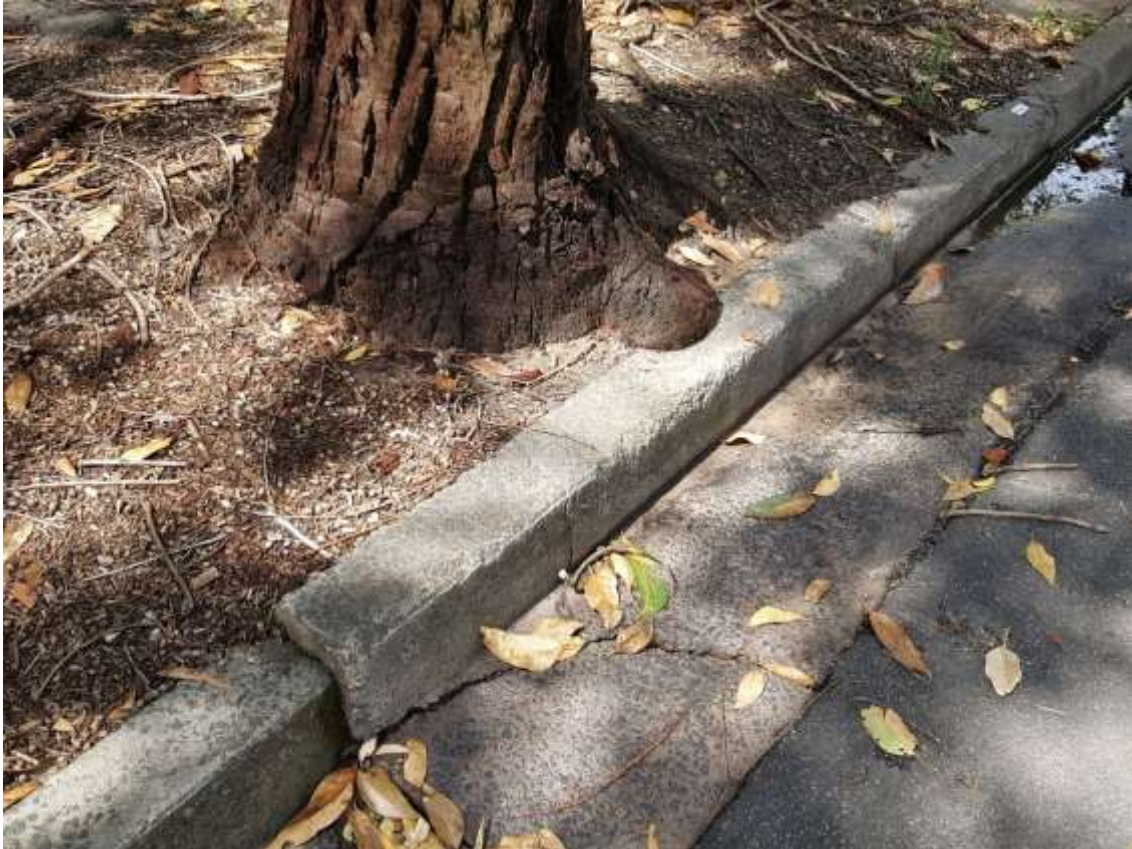
Photograph 9 – Tree 2 damage to kerb and gutter
