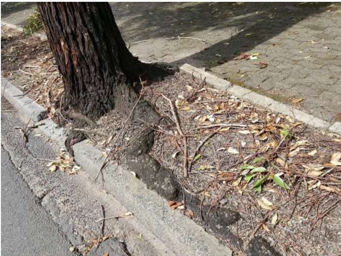
Photograph 20 – Tree 7 damage to kerb and gutter
