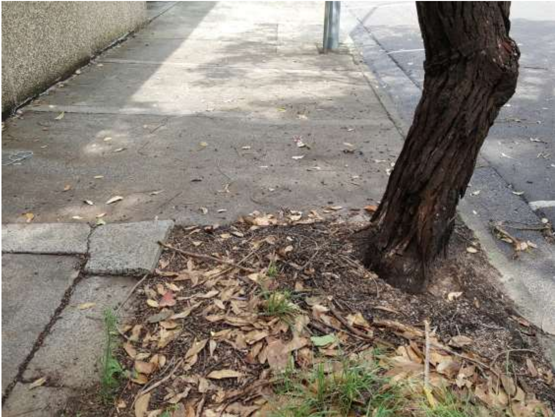
Photograph 3 – Tree 1 and adjacent damage to path
