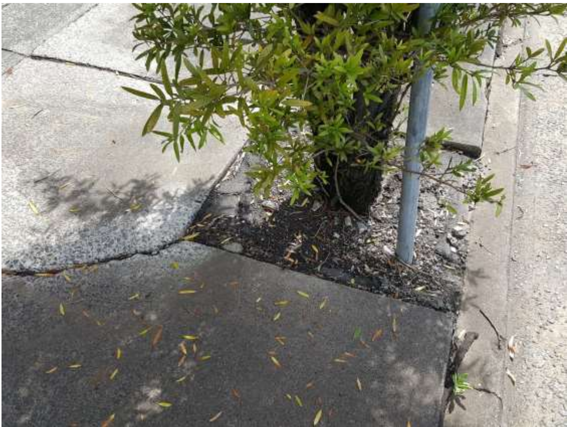
Photograph 26 – Tree 9 and adjacent damage to pavement
