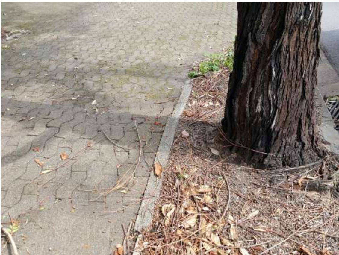
Photograph 16 – Tree 6 lifting of paved path
