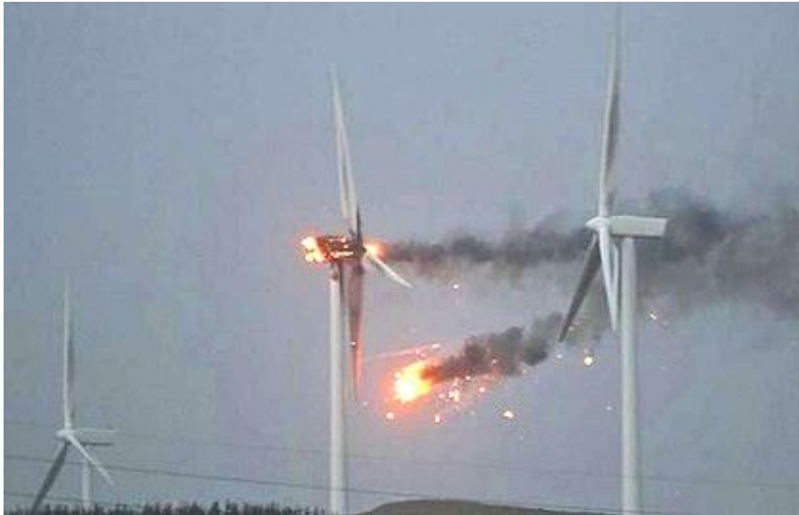
Figure 12.1 Wind turbine fire at nacelle. Caused by high wind conditions. Scotland, December 2011 Fires are difficult to extinguish due to the height of the turbine and the HazChem nature of the fire itself.
