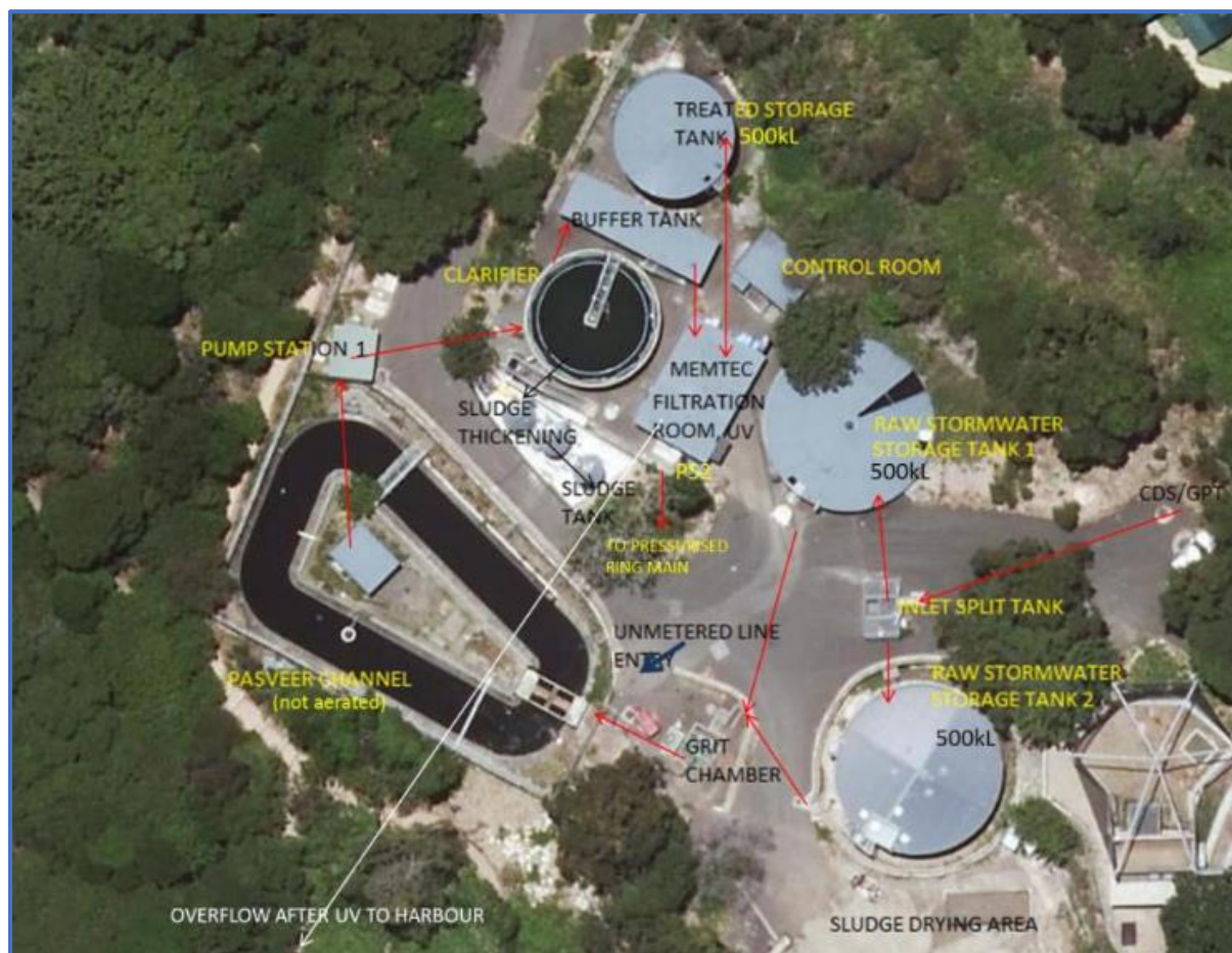
Figure 4.1 Waste Water Treatment Plant at Taronga Zoo
