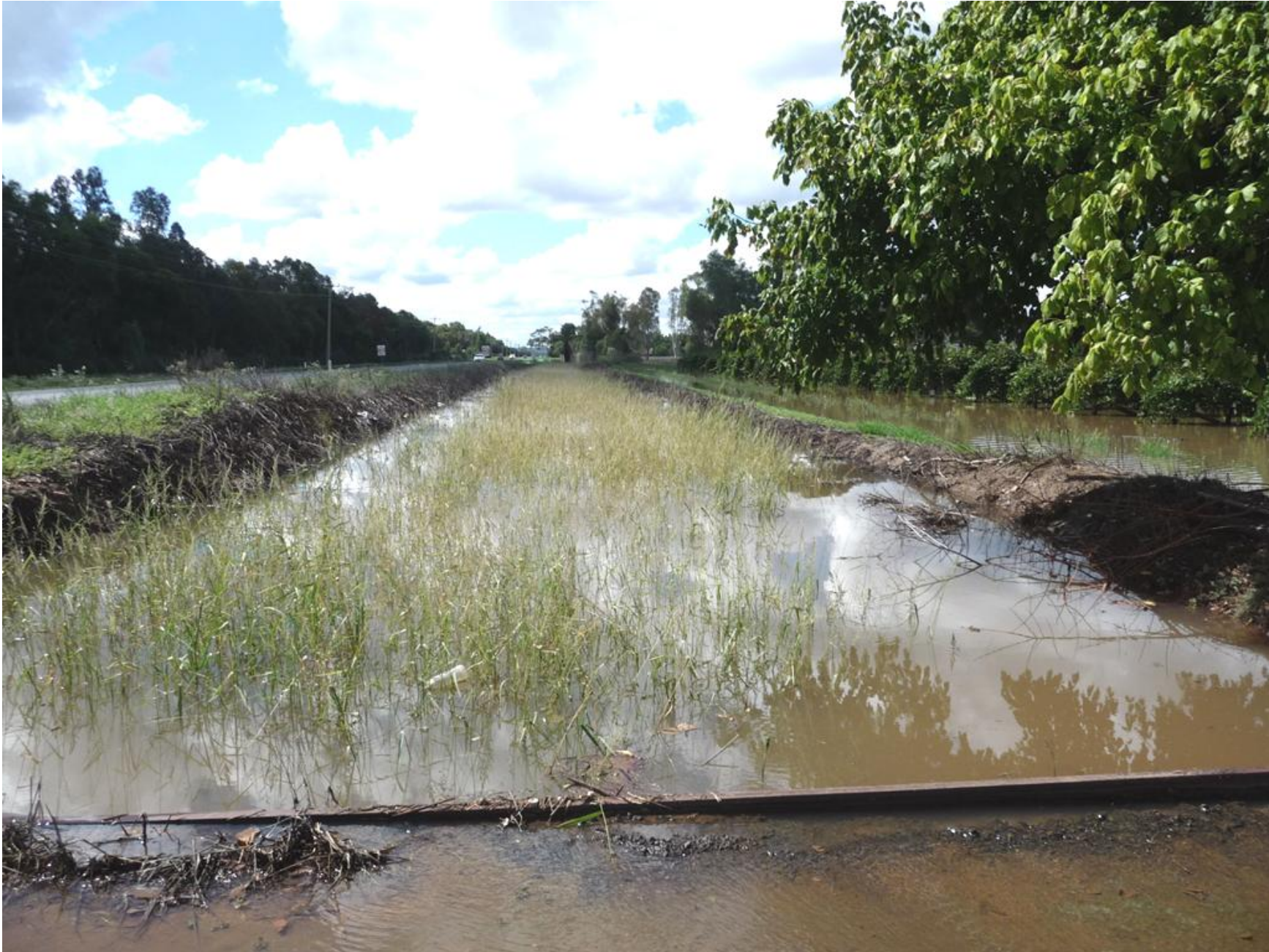
March 2012: MI drainage channel looking north towards Hanwood from Farm 132 Kidman Way entrance
