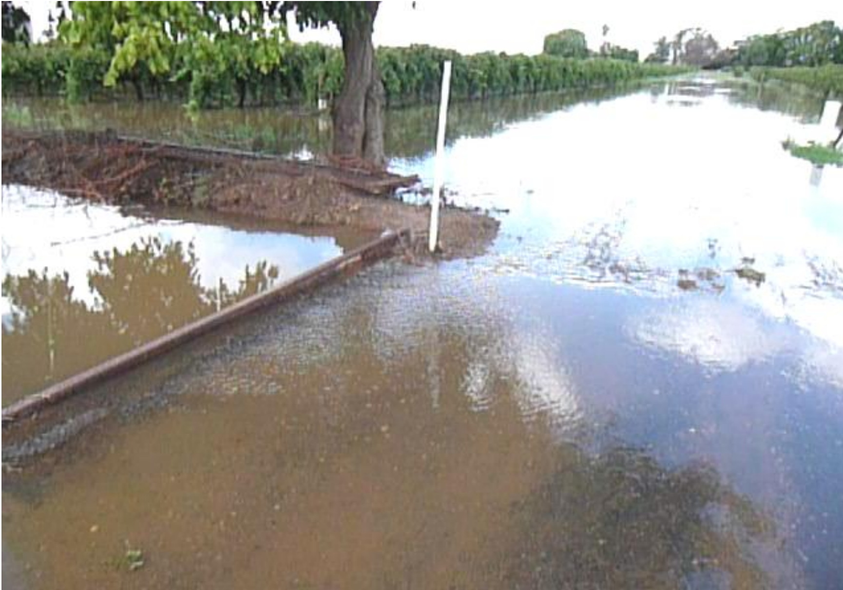
March 2012: Flooding from MI drainage channel into Farm 132 Kidman Way entrance
