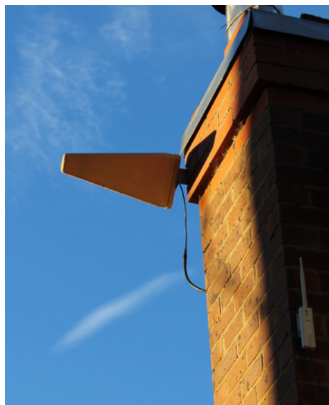
Figure 64: External antenna used for 4G Internet connection from J234A/B
