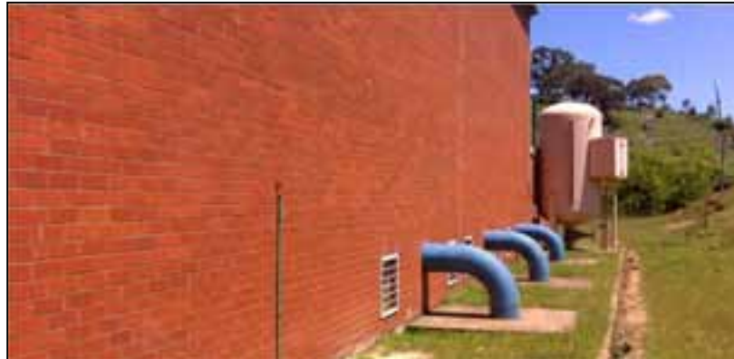
Figure 5-2: Suma Park Dam pumping station transfer main manifolds
