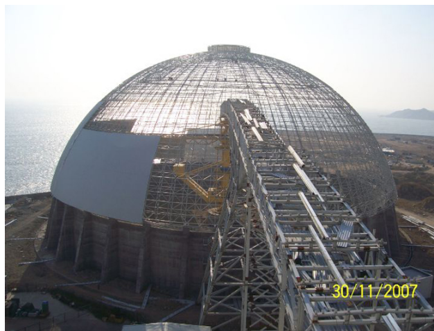
Figure 7: Construction of Coal Stockpile Building Huayang China
