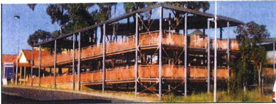
Figure 3: An example of a DDA compliant ramp for a 7.1m overpass
