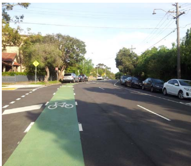
Figure 4 Example of On-Road Cycleway with Green Paint
